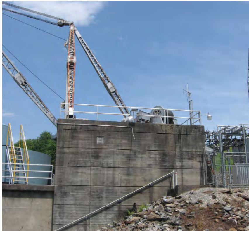
Figure 7: Chatuge Powerhouse, west elevation.
