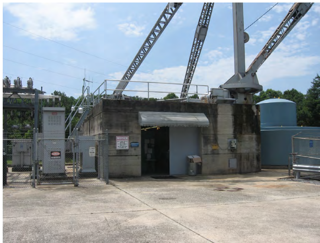
Figure 5: Chatuge Powerhouse, east elevation.
