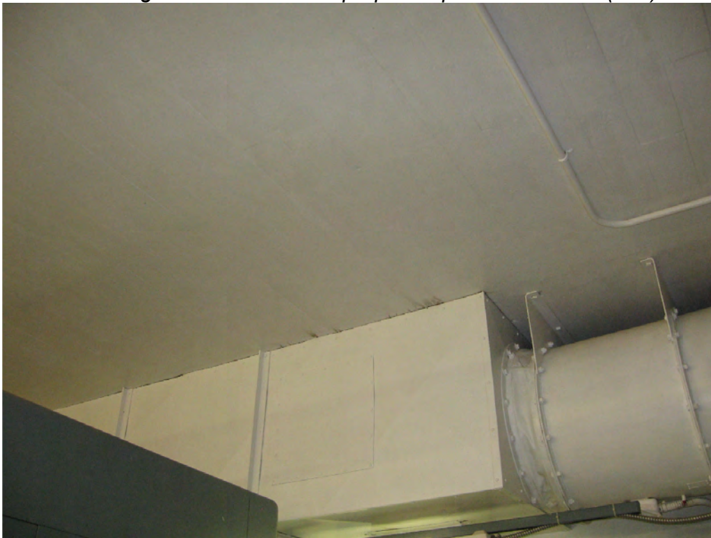
Figure 17: Interior of the powerhouse showing the location of the fixed camera at the ceiling which will monitor the main double doors leading into the control room.
