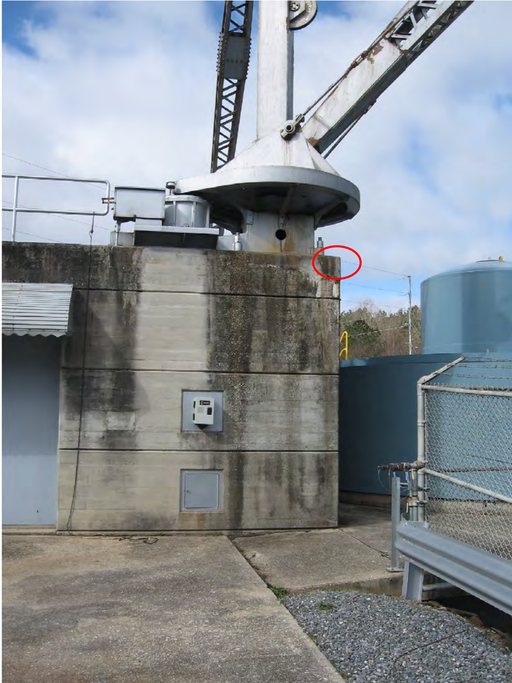
Figure 29: View of the powerhouse's east elevation showing the proposed location of a fixed camera at the building's northeast corner (red circle). This camera would monitor the control room double doors and the north and east elevations.
