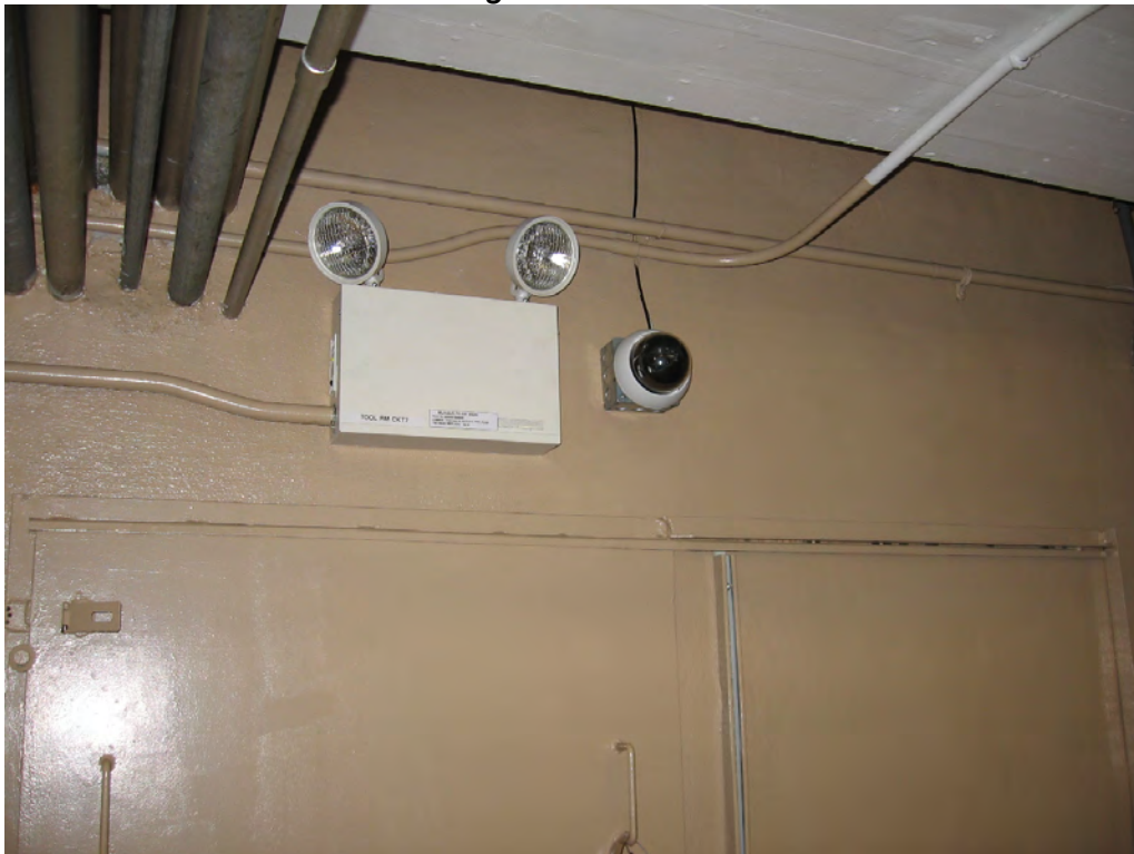
Figure 12: The new security cameras to be installed will be similar to this one wall-mounted camera at the Wilson Powerhouse in Alabama.
