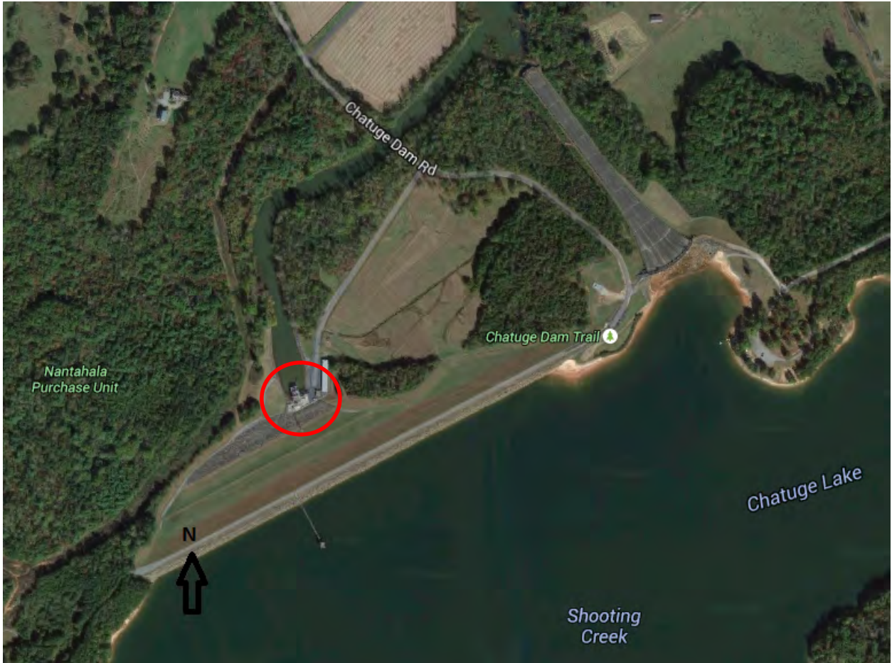
Figure 3: Aerial view of the Chatuge Hydroelectric Project. The red circle shows the location of the powerhouse.
