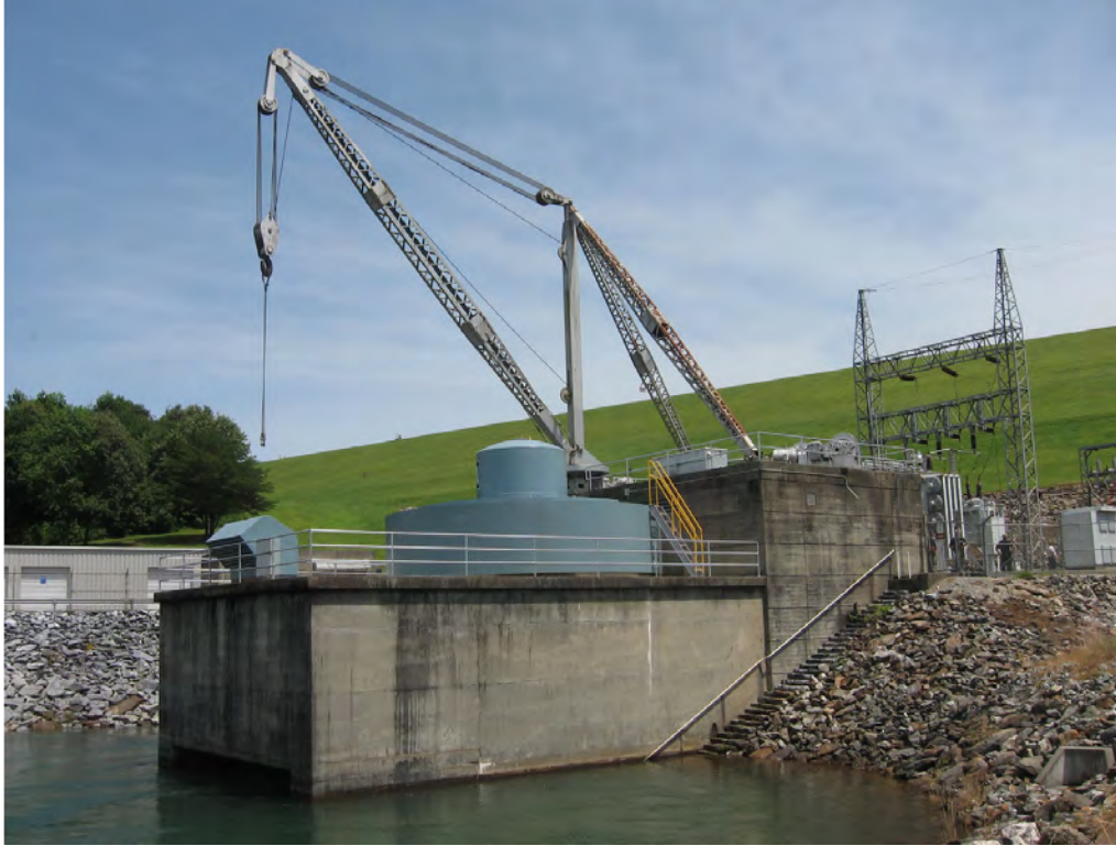
Figure 6: Chatuge Powerhouse, north and west elevations and adjacent switchyard.
