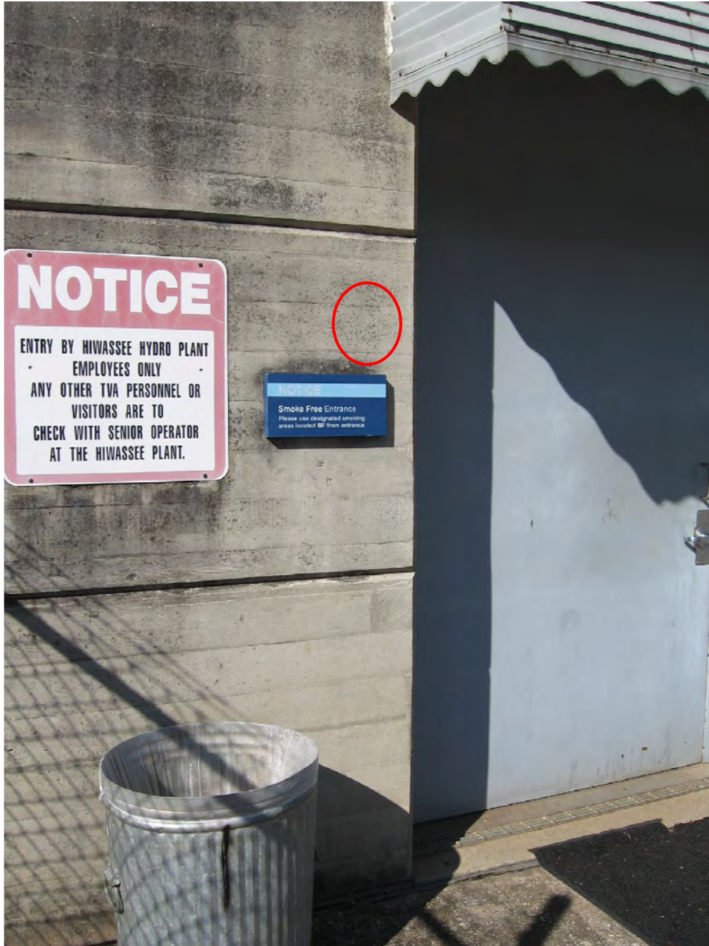
Figure 15: The location of the proposed card reader is shown as the red circle on the concrete wall adjacent to the main entrance to the control room on the east elevation of the powerhouse.
